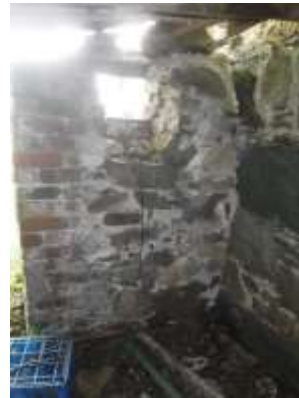
12 - inside of front wall to room 4
