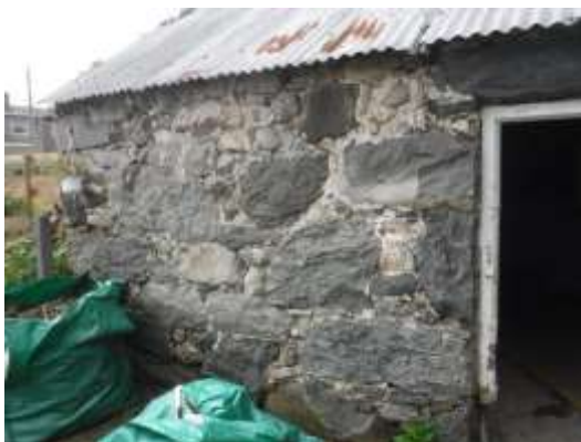
31 - front elevation to room 1 - large stones with smaller stone infill
