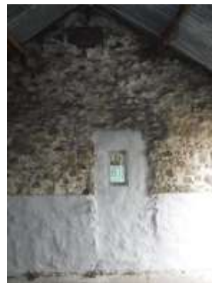
32 - wall between rooms 1 and 2, from room 1
