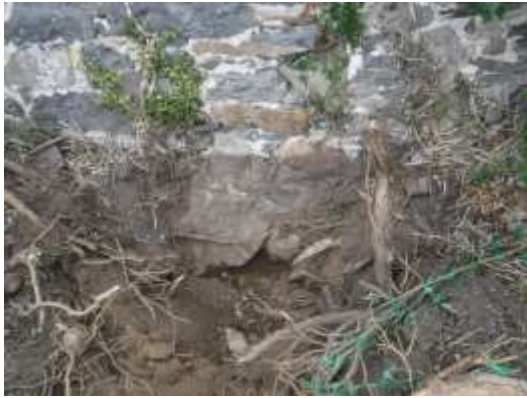
15 - south-east elevation - trial hole 1
