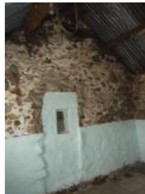
26 - wall between rooms 1 and 2, from room 2
