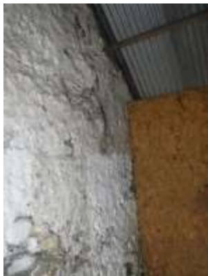
25 - wall between rooms 2 and 3, from room 3
