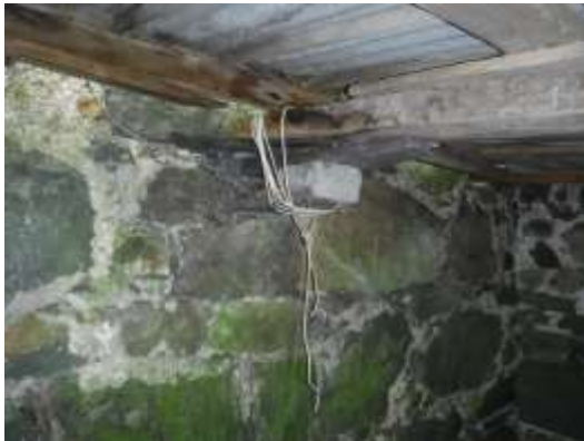
07 - temporary roof structure over room 4
