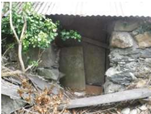
19 - rear elevation - temporary opening
