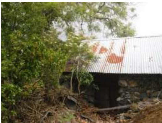
23 - junction of rear elevation and north-west gable - note adjacent tree
