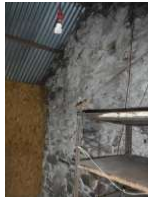
24 - wall between rooms 3 and 4, from room 3
