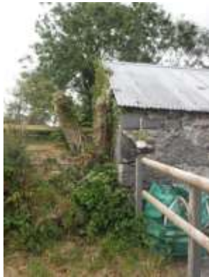
11 - tree located adjacent to south-east elevation
