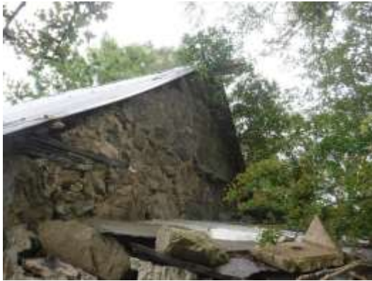
05 - gable pike to room 3
