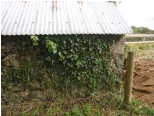
17 - rear elevation to room 1
